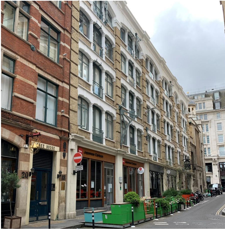
Figure 1: Historic Warehouses, Creechurch Lane
